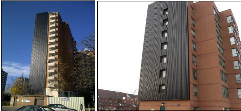
FIGURE 5 Solar Walls in two SHRRP projects in Toronto.
