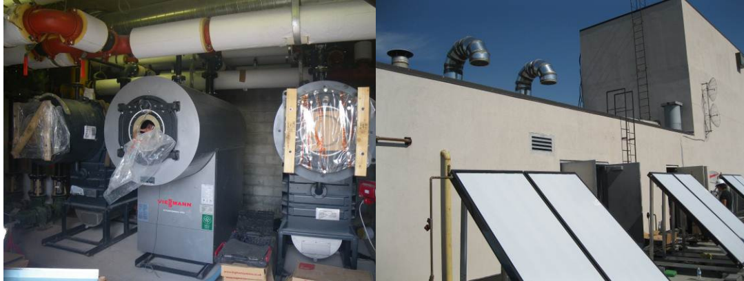
FIGURE 3 Major retrofits at Villa Otthon.
